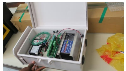
Re-inspection Re-inspection due to additional photo request from HU.
